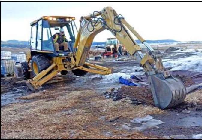
Removing hazardous waste at former wood treating facility, Lewistown (February 2016)
