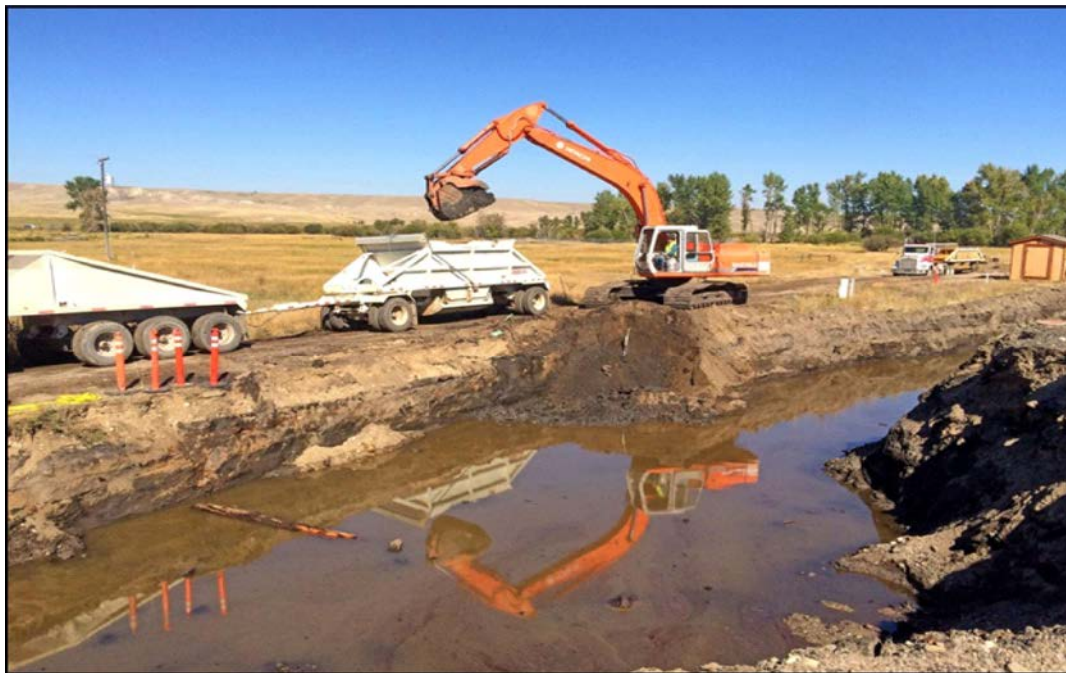
Excavating petroleum contamination at former Milwaukee Roundhouse facility in Deer Lodge (September 2015)
