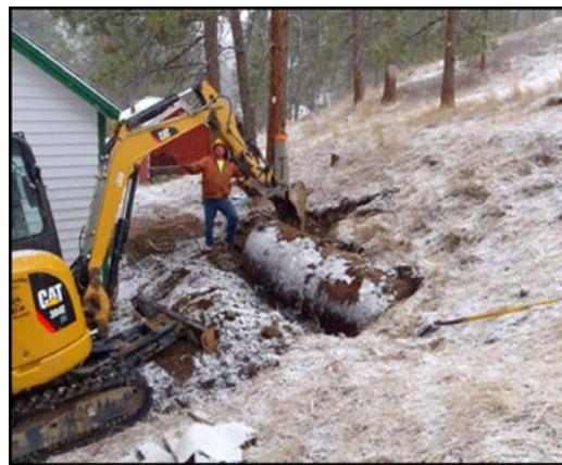
Removing half-buried tank at Unionville School (March 2016)
