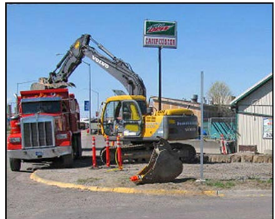
Excavating petroleum contaminated soil, Hardin (April 2016)
