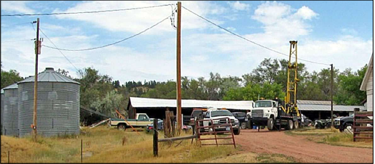
Drilling soil to verify cleanup of gasoline and diesel at rural farm near Decker (August 2016)
